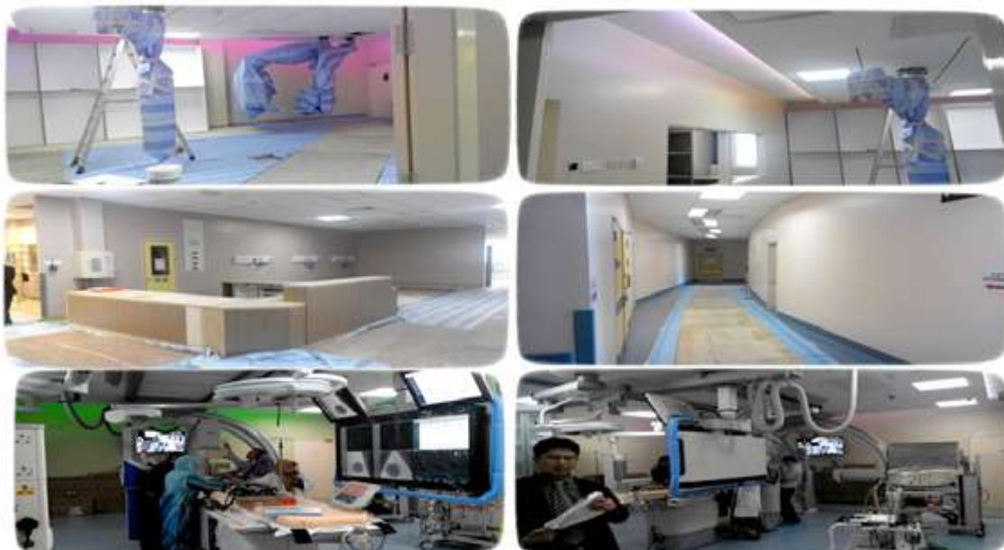
IMAGE 3 ICL PROJECT IN HOSPITAL SERDANG
